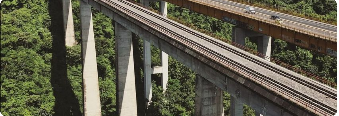
The Metlac Bridge, a landmark of the canyon and one of the most photographed engineering works in Veracruz.
